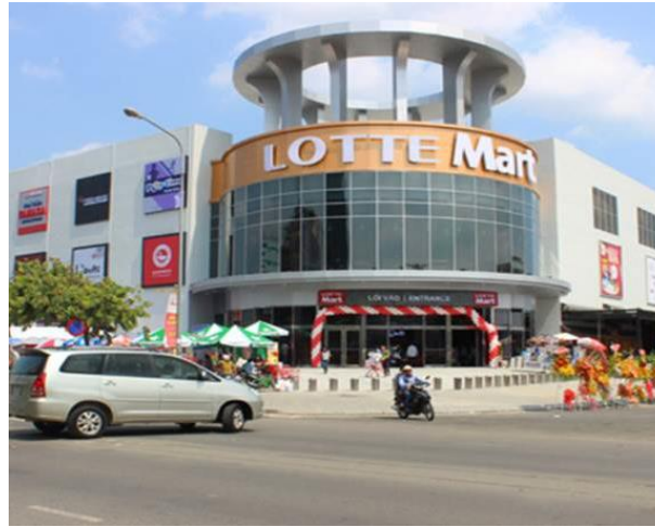
LOTTE MART Go Vap Jablotron security system Scale: floor 27,410m 2
