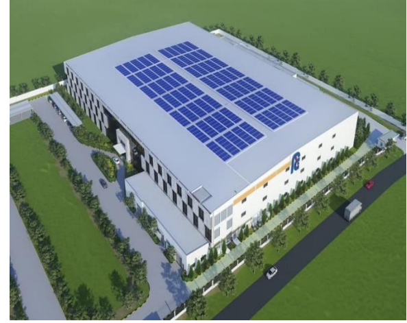
NEW APPAREL FAR EASTERN (Adidas) – VSIP BINH DUONG Security system Jablotron Scale of 55,000 m2
