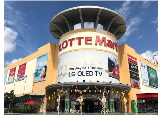
LOTTE MART Can Tho Jablotron security system Scale: 15,700m 2
