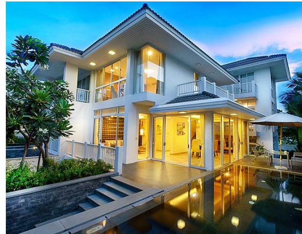
NGO QUANG HUY Villa Scale: 2 floors, 600m2 Jablotron alarm,
