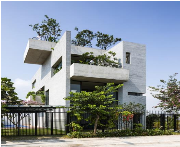
APARTMENT MR. NICOLAS – DISTRICT 9 Jablotron alarm
