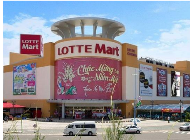
LOTTE MART Vung Tau Jablotron security system Scale: 23,501m 2
