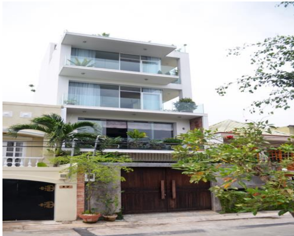
HOUSE OF CITY - HCM Security system and smart home
