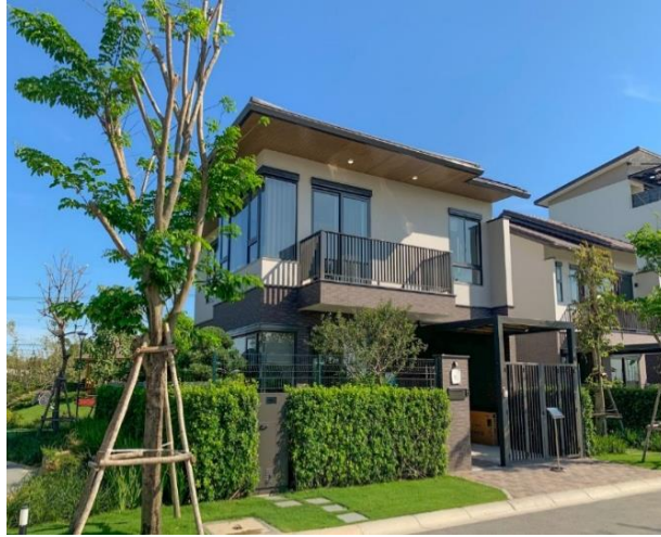
ANH PHUC VILLA - NHA TRANG Security system and smart home
