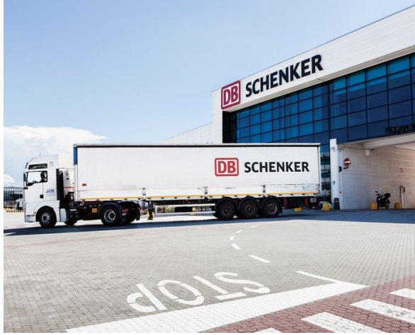
DB SCHENKER 1 Jablotron security system Scale: 1,500m2
