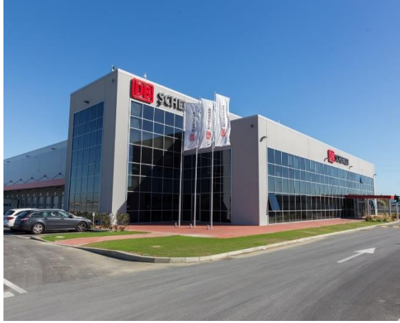
DB SCHENKER 2 Jablotron security system Scale: 3,000m2
