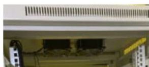
Fan units for dissipate heat
