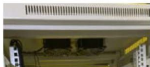
Fan units for dissipate heat
